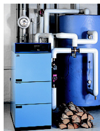
Baxi log boiler and accumulator tank
